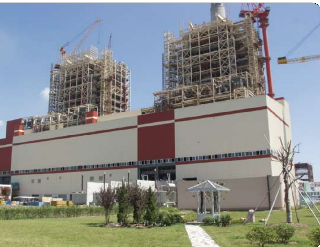
Wai GaoQiao coal power station near completion
