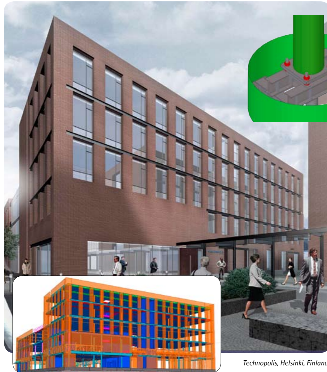
Steel foundation that can support two floors of the building before casting the concrete for the foundation (Technopolis, Helsinki, Finland). Steel foundation is a new product concept of Finnish Rautaruukki Oyj, and piloted for the first time in Technopolis.
